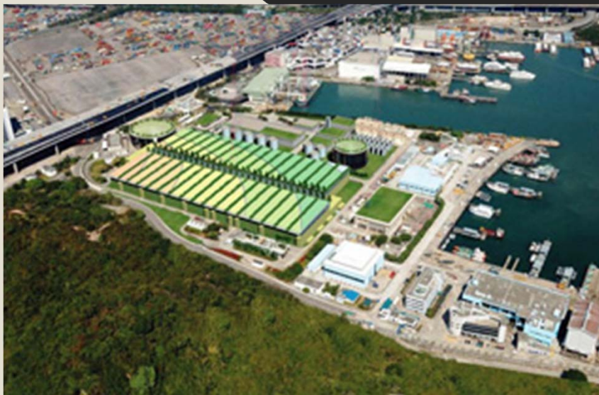
Stone Cutter's Island Treatment Plant
